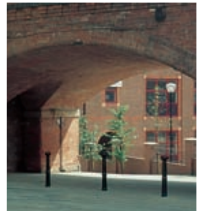
A new link has been punched through the railway viaduct - helping to stitch together the city centre and riverfront
