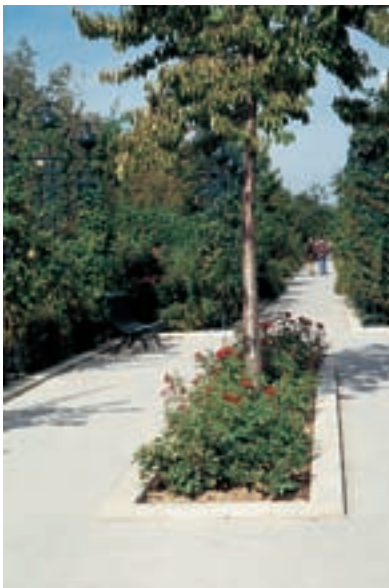
A linear park of exceptional quality runs along the top of the viaduct.
