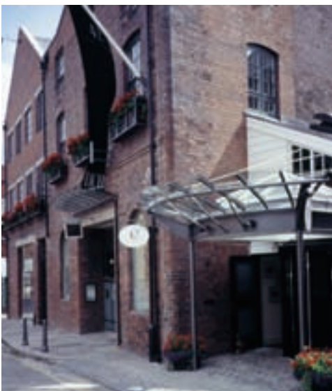
High quality architecture has raised design standards in the area
