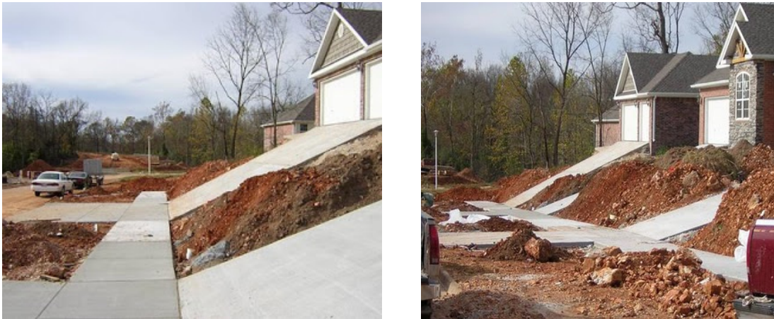
Figure F-14 (Pictures of a Poor Grading Design on a Residential Project)
