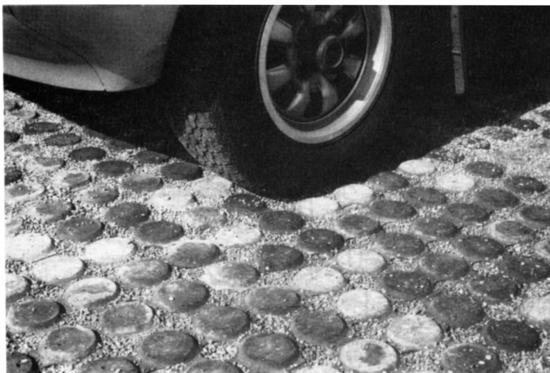
Fig. 8. Surface detail on experimental permeable pavement
