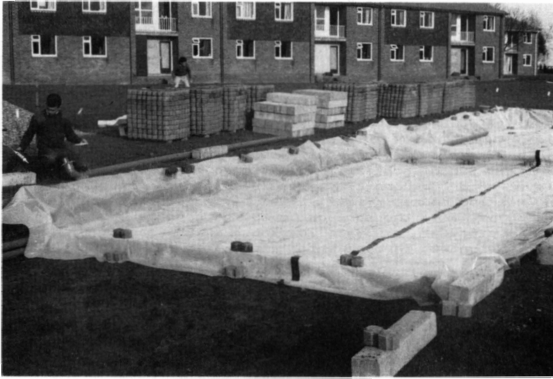
Fig. 2. Experimental permeable pavement construction showing impermeable membrane on formation
